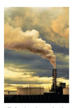
▲ The flow of gases from a smokestack can be measured by releasing <sup>41</sup>Ar and monitoring its passage.
