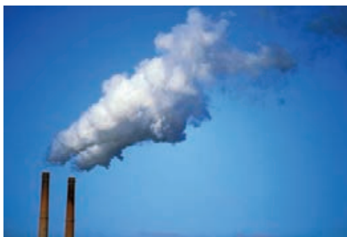
Figure 6.9 | Water is a product of the combustion of hydrocarbons. Here we see clouds of condensed water vapor coming from the stacks of an oil-fired electric generating plant during the winter. (PictureNet/©Corbis)
