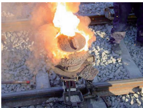
Figure 4.5 | The thermite reaction. Pictured here is a device for making white-hot iron by the reaction of aluminum with iron oxide and letting the molten iron run down into a mold between ends of two steel railroad rails. This welds the rails together. (Wikimedia Commons)
