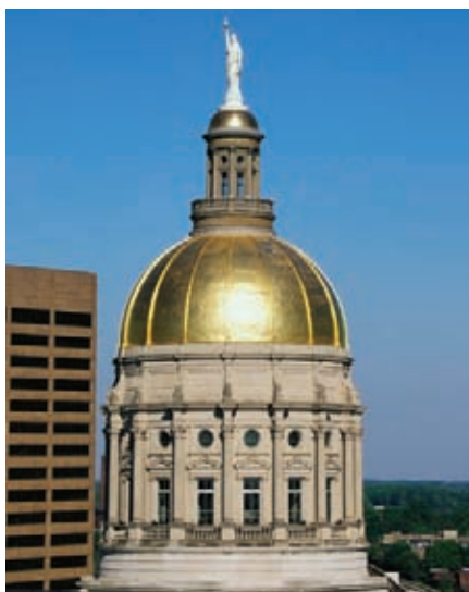
Figure 3.10 | Malleability of gold. Pure gold is not usually used in jewelry because it is too malleable. It is used decoratively to cover domes since it can be hammered into very thin sheets called gold leaf. (Joseph Sohm; Visions of America/©Corbis)
